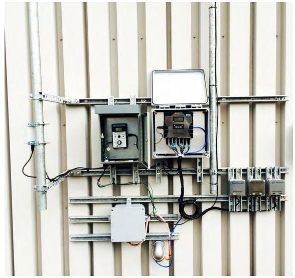
Full Installation – Note the magnetometer on brackets extended off building (far left)
